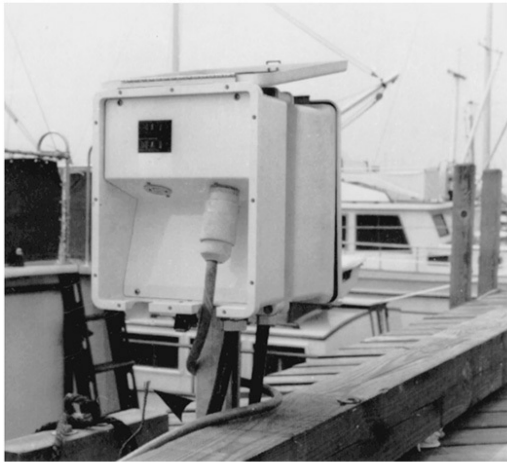
Fig. 555-4. Receptacle providing shore power to each boat is contained in a “power pedestal” and is a locking and grounding type. (Sec. 555.19.)
