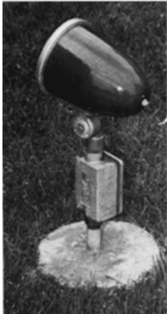
Fig. 314-28. A single rigid metal conduit may not support a box, even with concrete fill in the ground (left). Box may not be supported on EMT, even with several connections used (center). Method at right is a violation on three counts: EMT, not “conduit,” supports the box; only one hub on box is connected; box is more than 18 in. above ground. (Sec. 314.23.)
