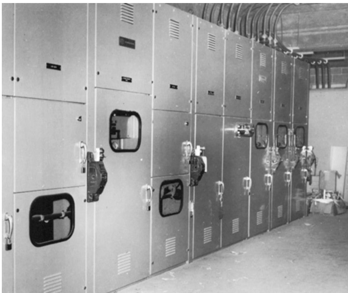
Fig. 490-12. Load-interrupter switchgear is generally used with fuses to provide protection as well as load-break switching for medium-voltage circuits. The fuses must be rated to provide complete protection for the load interrupter on closing, carrying, or interrupting current—up to the assigned maximum short-circuit rating. (Sec. 490.21.)
