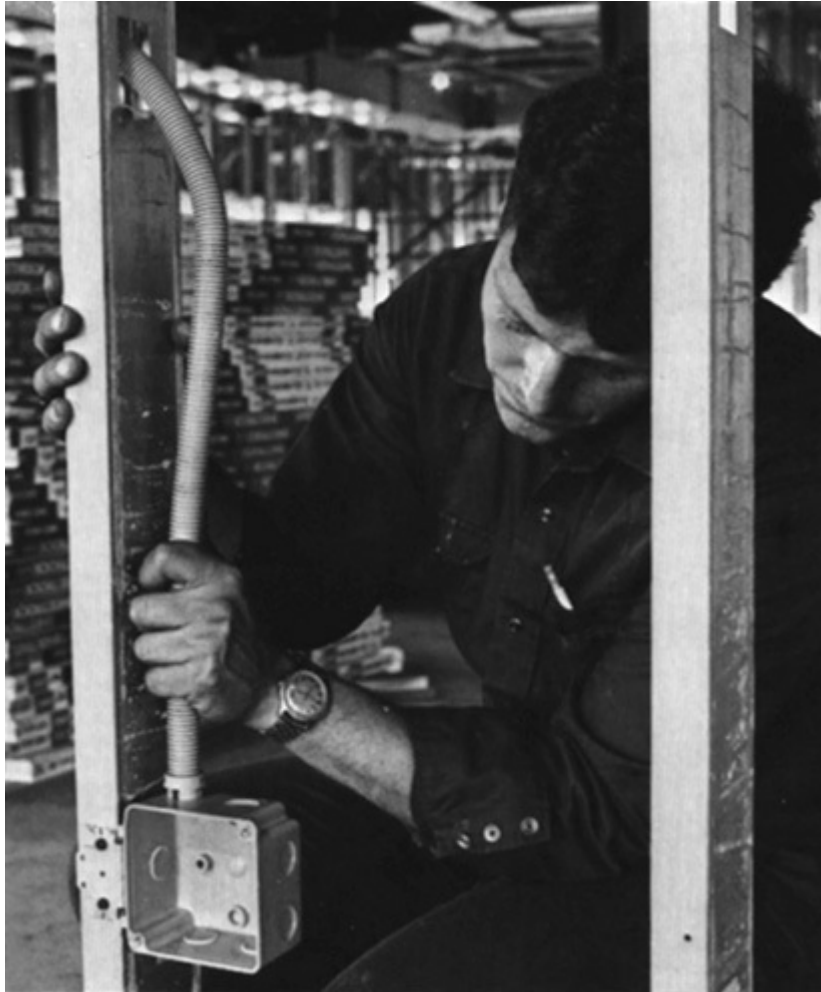
Fig. 362-1. ENT is a pliable, bendable plastic raceway for general-purpose use for feeders and branch circuits.
