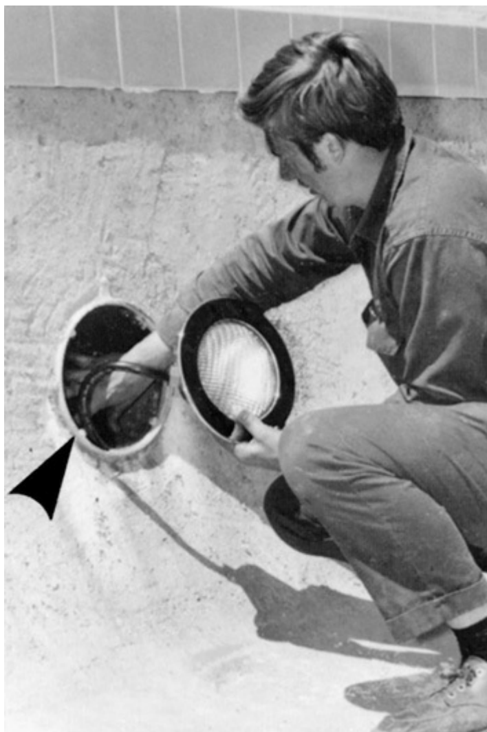
Fig. 680-3. Wet-niche luminaire consists of forming shell set in pool wall with cord-connected lamp-and-lens assembly that attaches to the forming shell, with cord coiled within the shell housing. (Sec. 680.2.)
