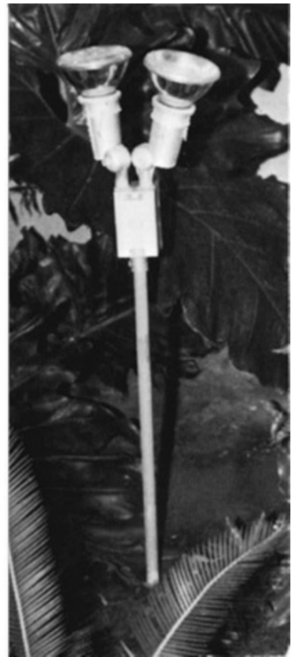
Fig. 314-28. A single rigid metal conduit may not support a box, even with concrete fill in the ground (left). Box may not be supported on EMT, even with several connections used (center). Method at right is a violation on three counts: EMT, not “conduit,” supports the box; only one hub on box is connected; box is more than 18 in. above ground. (Sec. 314.23.)
