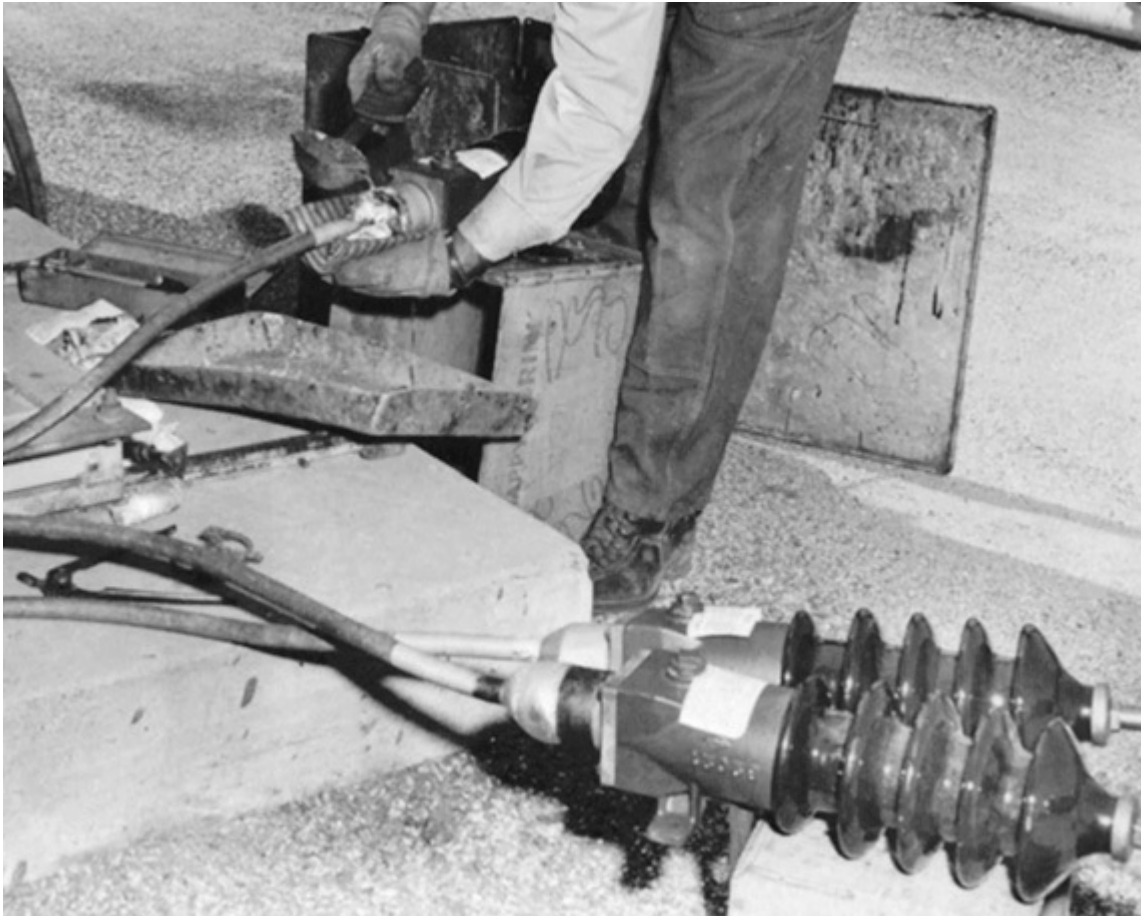
Fig. 300-56. A pothead is used on the end of each paper-insulated, lead-covered cable to protect against entry of moisture, with a wiped lead joint at the terminal. (Sec. 300.42.)
