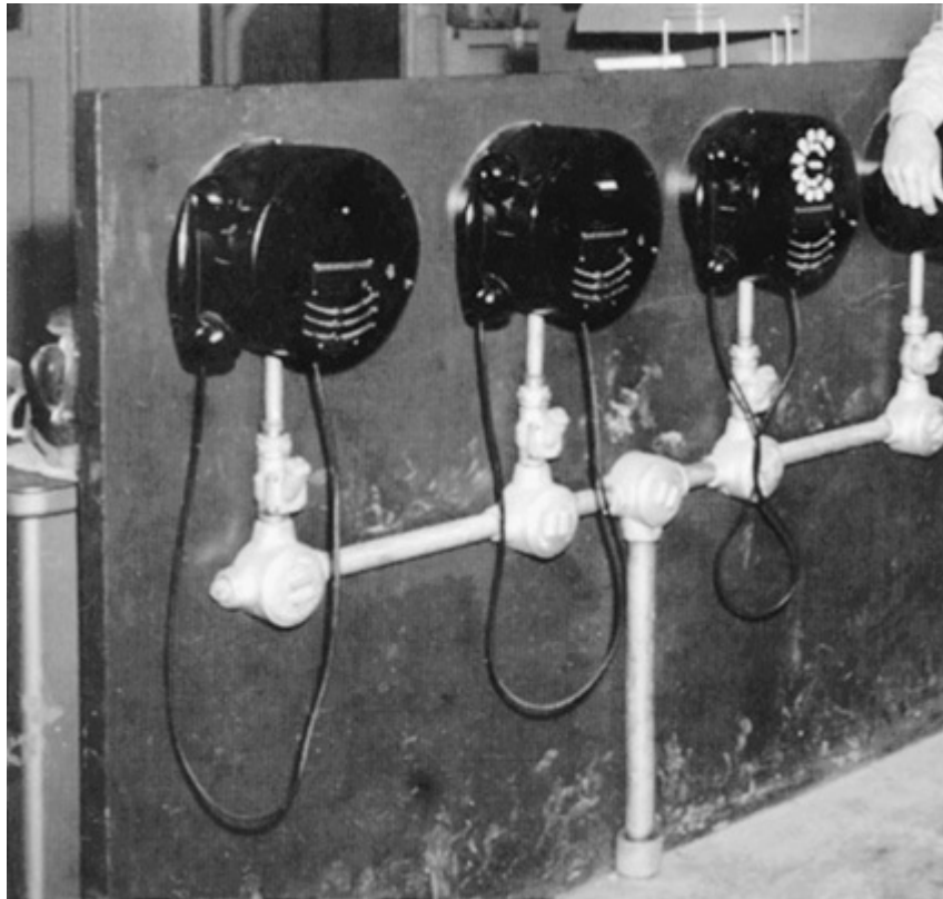
Fig. 501-40. Explosionproof telephones are made and listed for Class I, Groups B, C, and D, and must be connected with the necessary seal fittings required in conduits to enclosures housing arcing or sparking devices. [Sec. 501.150(4).]
