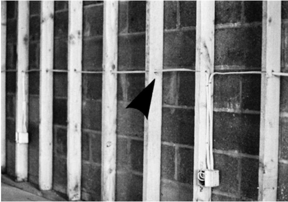
Fig. 334-7. NM or NMC cables must be stapled every 4½ ft (1.4 m) where attached to the surfaces of studs, joints, and other wood structural members. It is not necessary to use staples or straps on runs that are supported by the drilled holes through which the cable is pulled. But there must be a staple within 12 in. (300 mm) of every box or enclosure in which the cable terminates. This illustrates the distinction between support intervals, which the stud drillings provide, and securement, which only the staples provide. Cable ties, if listed for “securement and support,” are also permitted; their usual application is above suspended ceilings. (Sec. 334.30.)
