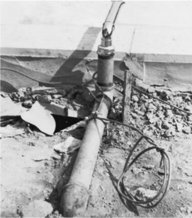
Fig. 680-17. Water-fill pipe and metal housings associated with the water-circulation system are “bonded” with an 8 AWG solid copper conductor, as required. (Sec. 680.26.)
