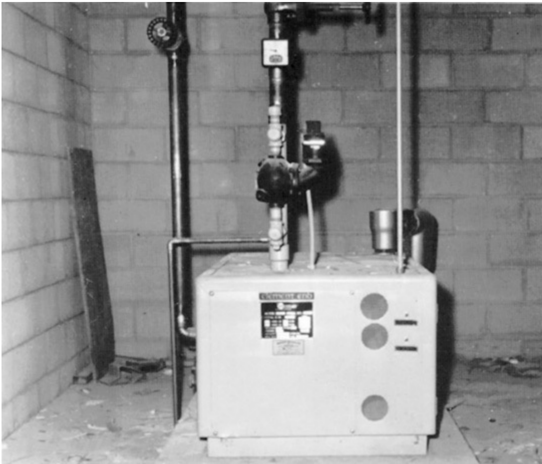
Fig. 424-17. Electric boilers with resistance-type heating elements are regulated by Secs. 424.70 through 424.74. (Sec. 424.70.)
