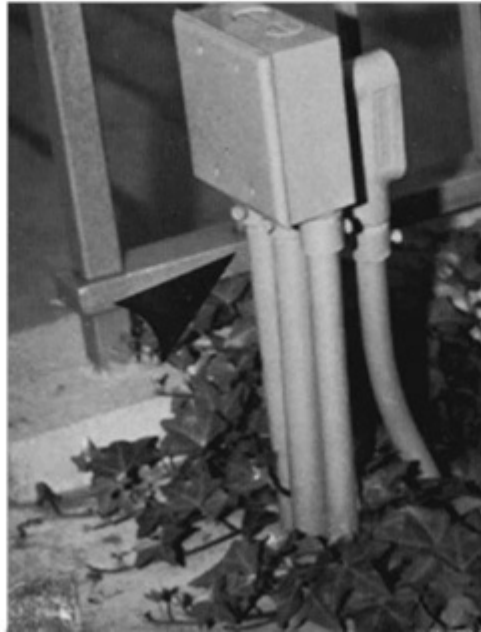
Fig. 314-28. A single rigid metal conduit may not support a box, even with concrete fill in the ground (left). Box may not be supported on EMT, even with several connections used (center). Method at right is a violation on three counts: EMT, not “conduit,” supports the box; only one hub on box is connected; box is more than 18 in. above ground. (Sec. 314.23.)
