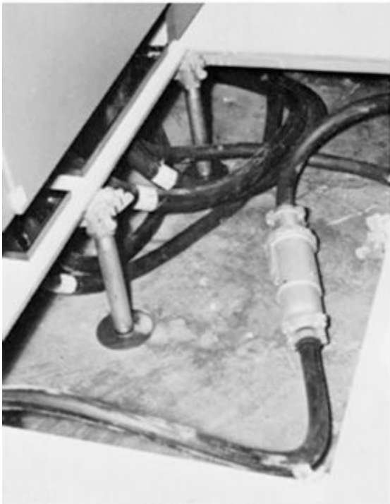
Fig. 645-1. Connection of data-processing units to their supply circuits and interconnection between units (power supply, memory storage, etc.) may be made only with cables or cord-sets specifically listed [see (B)(2)] as parts of the data processing system. (Sec. 645.5.)
