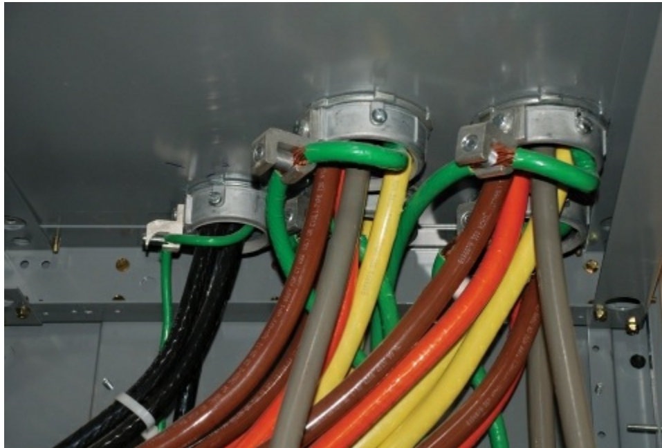
Figure 9.7 MC cable that provides an equipment grounding conductor (wire-type) in the assembly, and the sheath is suitable as an equipment grounding conductor. Courtesy of Southwire Company
