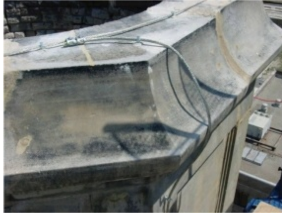
Photo 21.9 Example of a proper down conductor bend radius Courtesy of Guardian Equipment Company of Novi, MI
