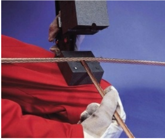
Photo 7.3 Wires placed in mold
