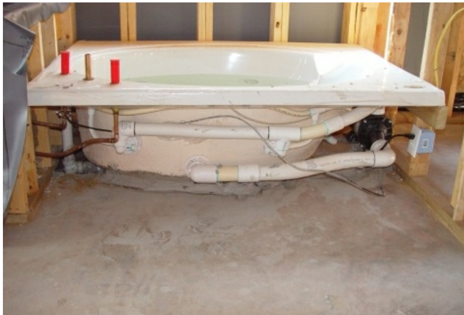
Photo 16.11 bonding of hydromassage bathtubs
