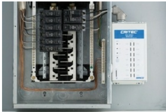
Photo 21.14 Installation of surge protection on incoming service Courtesy of Erico
