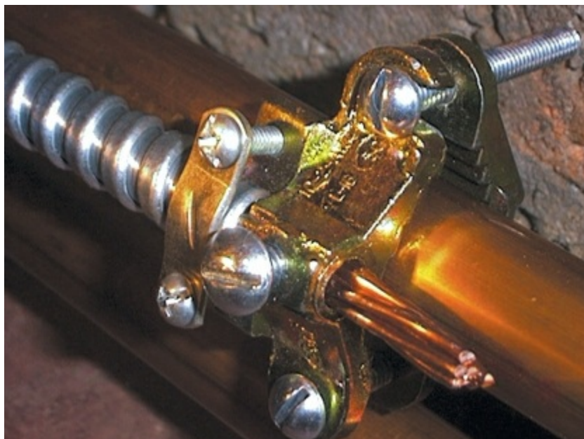
Photo 7.14 Grounding electrode conductor bonded to conduit with jumper same size as grounding electrode conductor
