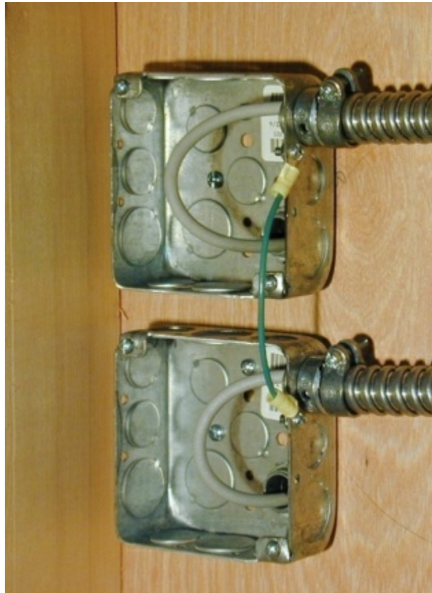
Photo 16.3 Metal parts bonded together using equipment suitable for the use
