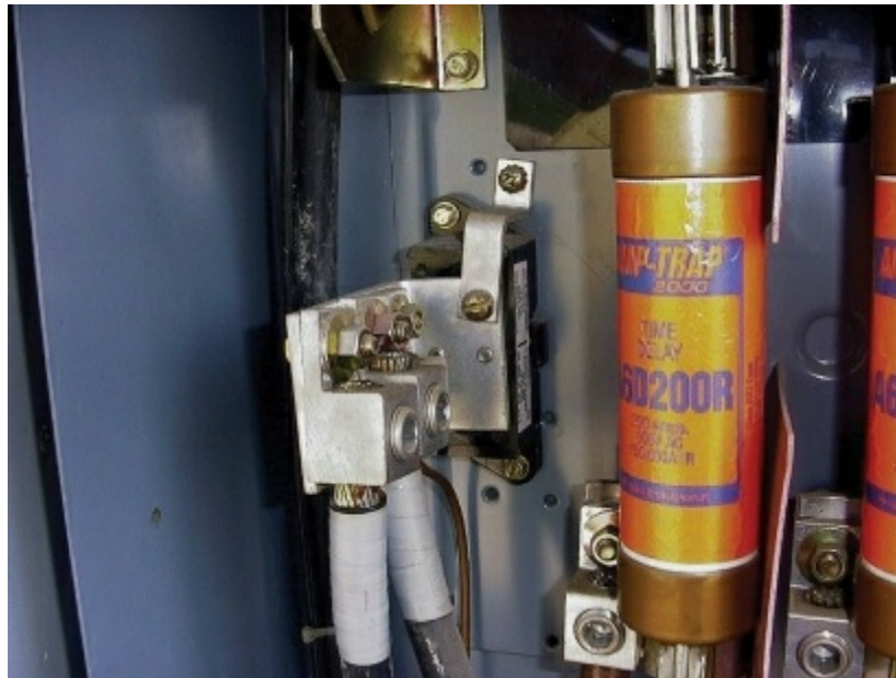
Photo 5.1 Main bonding jumper (strap type)
