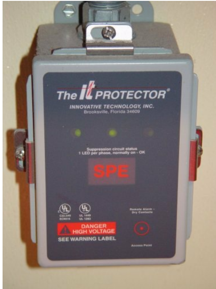
Photo 18.6 Typical three-phase surge protective device (SPD)
