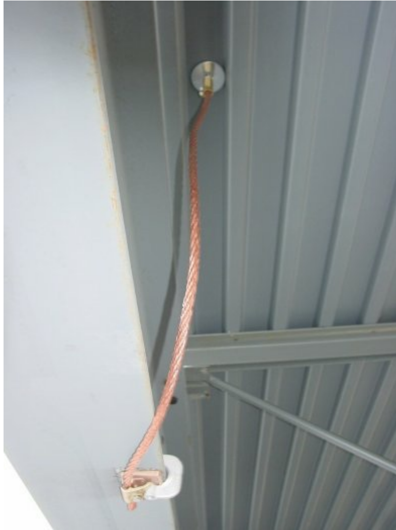
Photo 21.10 Example of interior connections to the steel frame from the through-roof connector Courtesy of Guardian Equipment Company of Novi, MI
