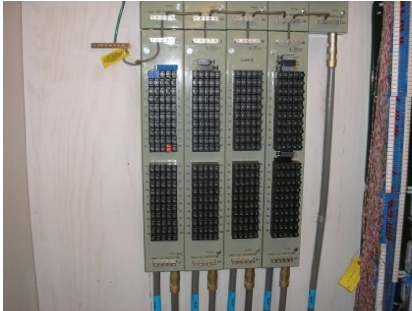
Photo 21.15 Installation of surge protection on communication lines at the service entry
