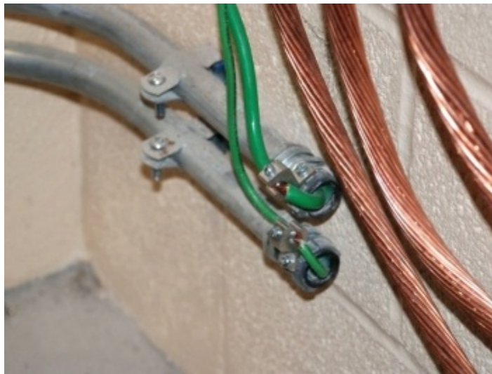
Photo 7.14 Grounding electrode conductor bonded to conduit with jumper same size as grounding electrode conductor
