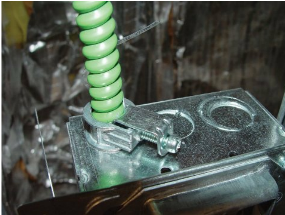
Photo 9.5 Installation of AC cable that is acceptable for use in patient care areas because it provides two equipment grounding conductor paths (sheath and conductor)
