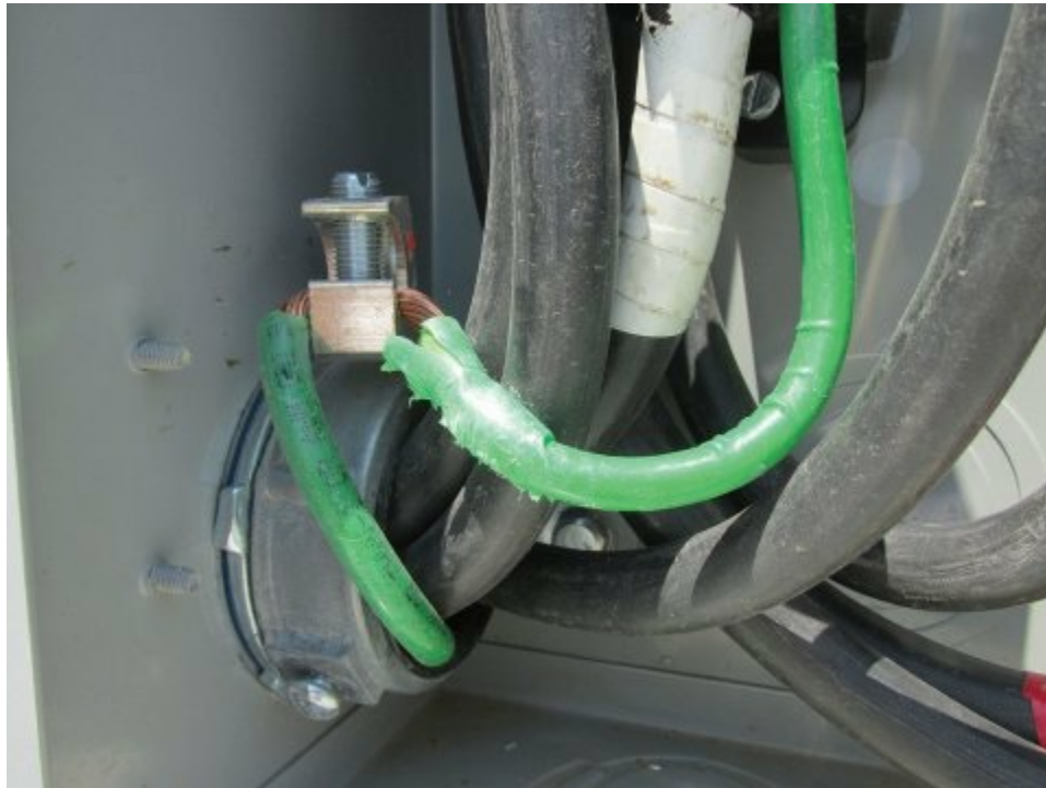
Photo 5.4 Grounding (bonding) bushing for use in bonding on the supply side of service disconnect
