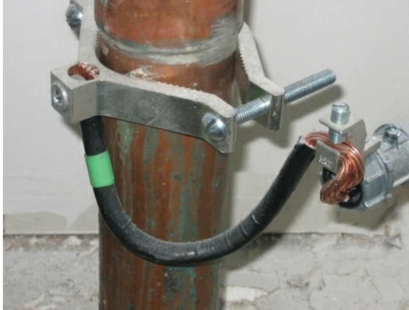
Photo 8.9 Connection to water piping is to be accessible.
