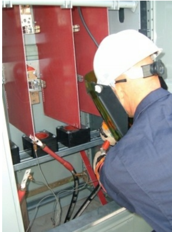
PHOTO 1.1 Insulation-resistance (hi-potential) testing in progress. Courtesy of Electro-Test, Inc.
