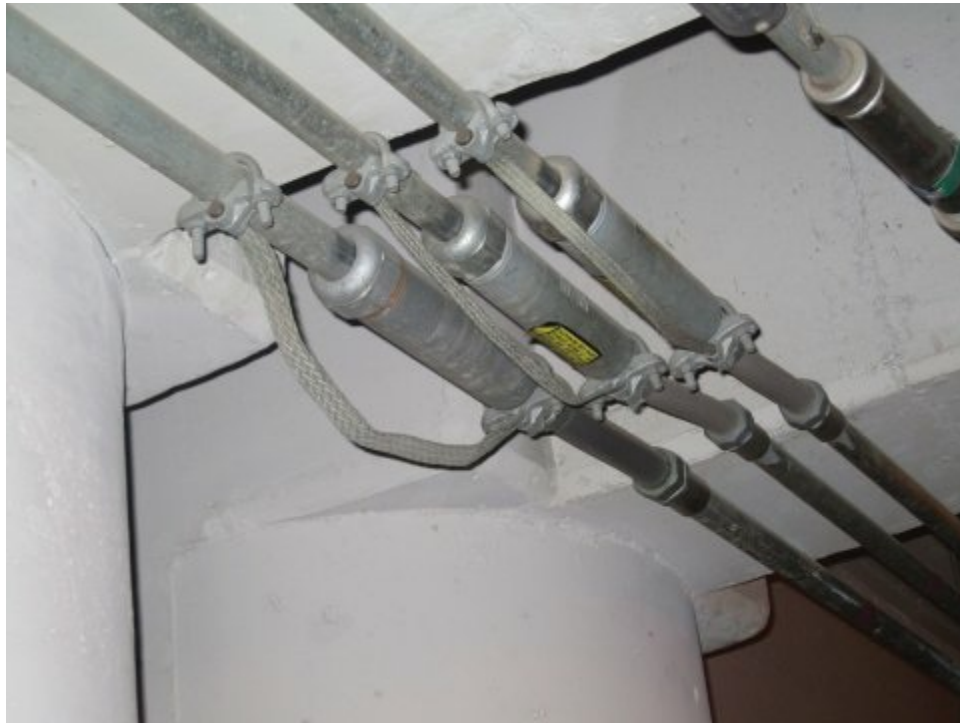
Photo 8.3 Expansion coupling
