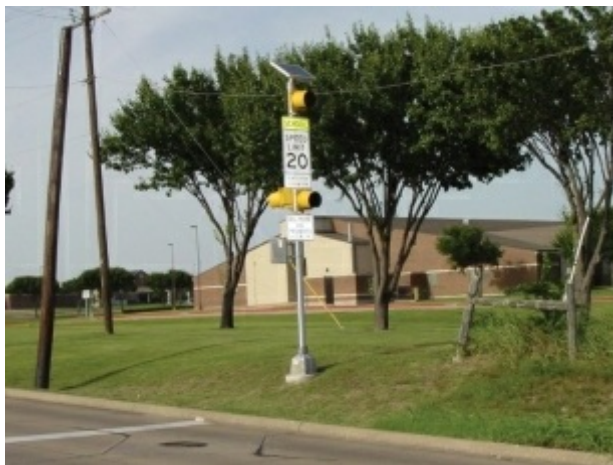
Photo 17.1 PV-powered school zone sign
