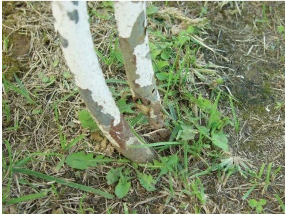
Photo 9.8 Metal raceway that has been severely damaged due to corrosion
