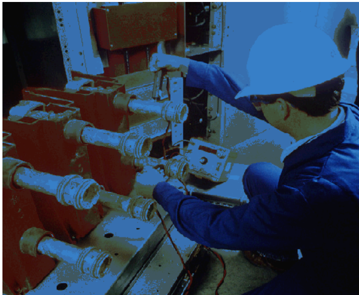
Figure 6-3—Contact resistance testing
