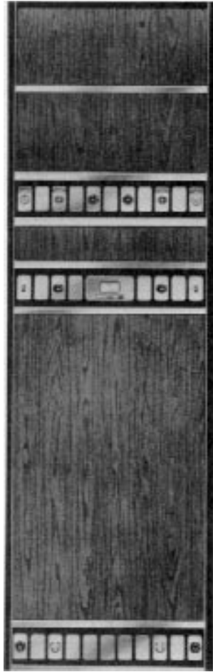
Figure 4-4—Full single-section general care wall
