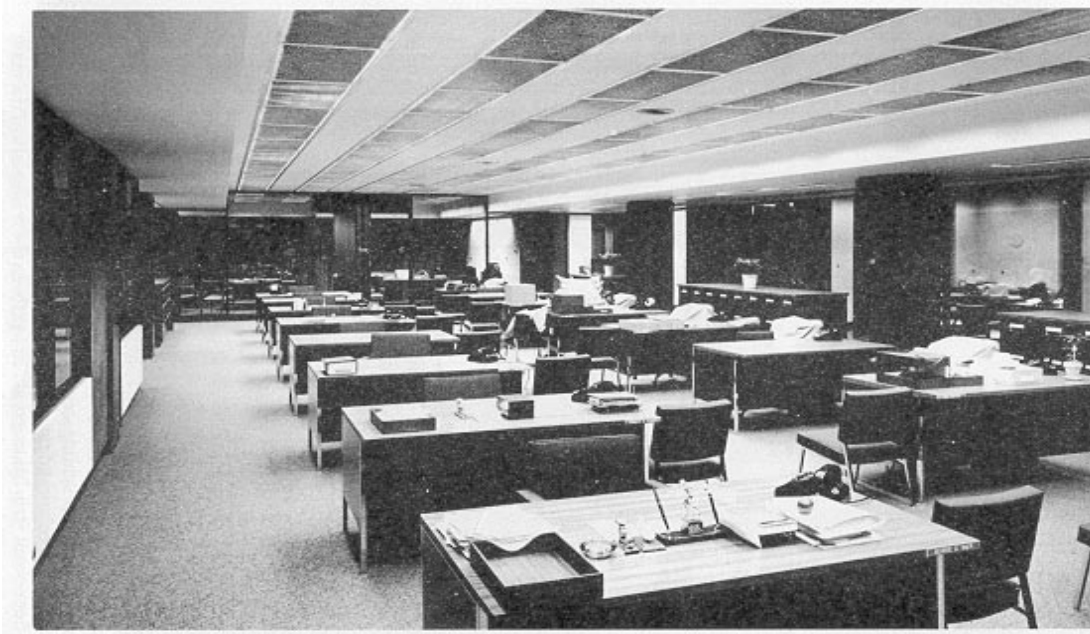
Figure 135—Parabolic Wedge Louver
