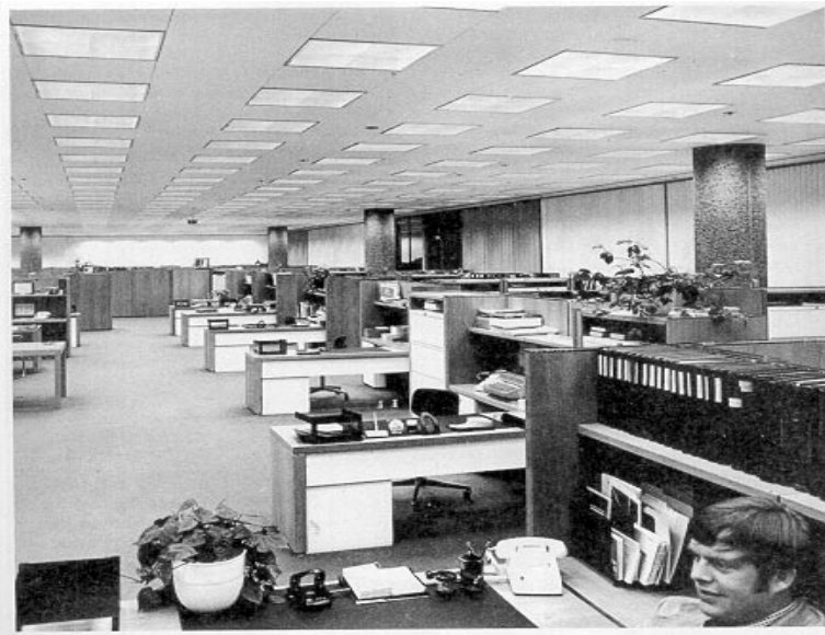
Figure 128—Two U-Shaped Fluorescent Lamps, with Efficient, Low-Brightness Anodized Aluminum Luminaire, Are Employed in Each Unit to Supply Lighting from the Ceiling
